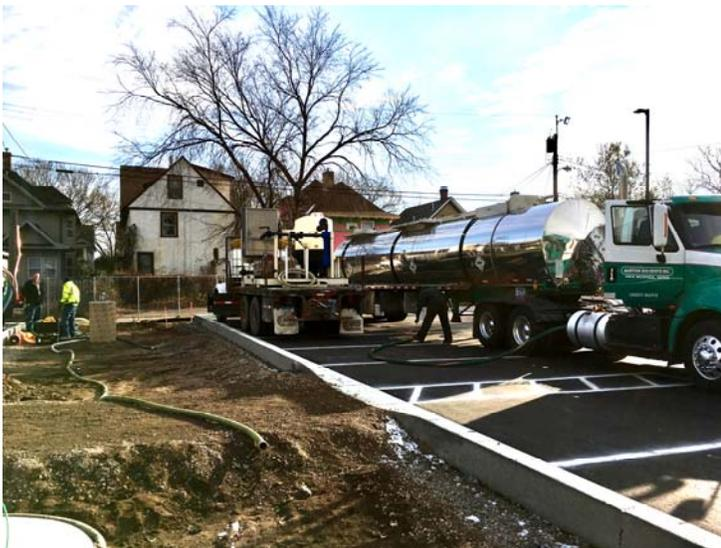
*The large tank truck is filled with deionized water and glycol. The other truck has all the pumps and valves. Together, they are giving the geothermal wells their final fill. The guys operating them are taking great pains to make sure there is not one air bubble in the system!*
