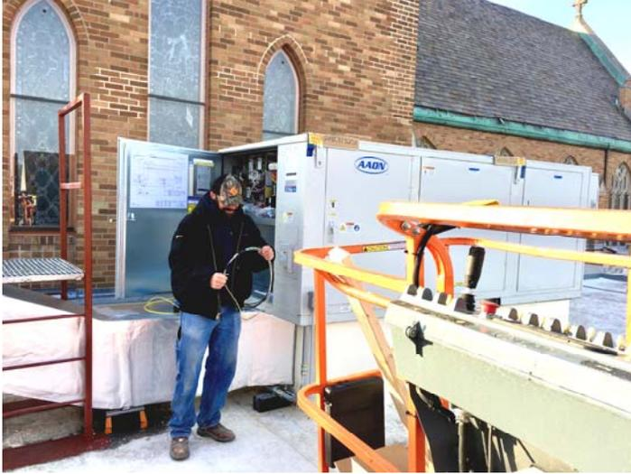
*The big machine is the fresh air unit on the Parish House roof. This exchanges inside stale air for healthy outside air. Electrician Tony is trying to figure out where all those mysterious wires need to go (he really knows; he was just looking very serious for the camera.).*
