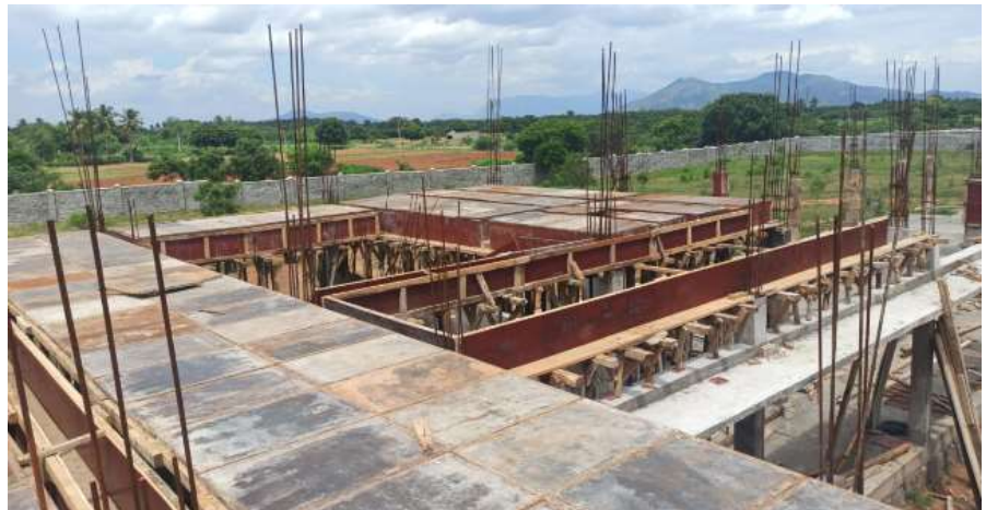
The Shalom Home now under construction.
